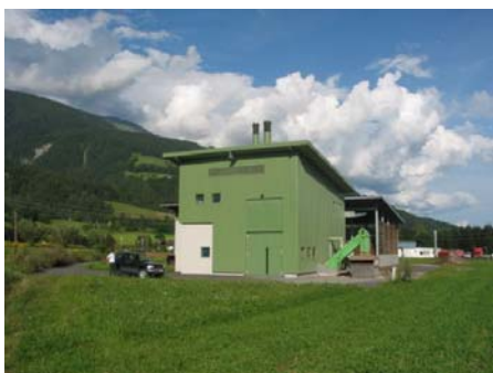
One of three biomass district heating plants
