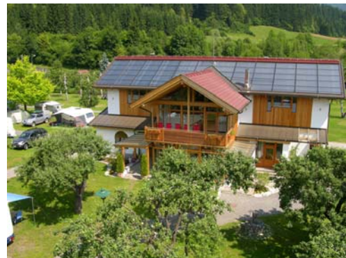
Campsite Alpengcamp with bio demonstration heating system
